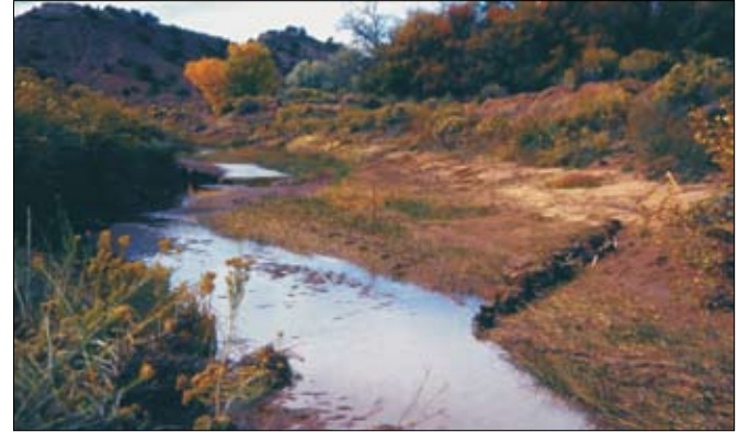
Point bar evolving downstream of properly installed post vane with trimmed posts. (Photo courtesy of Bill Zeedyk.)
